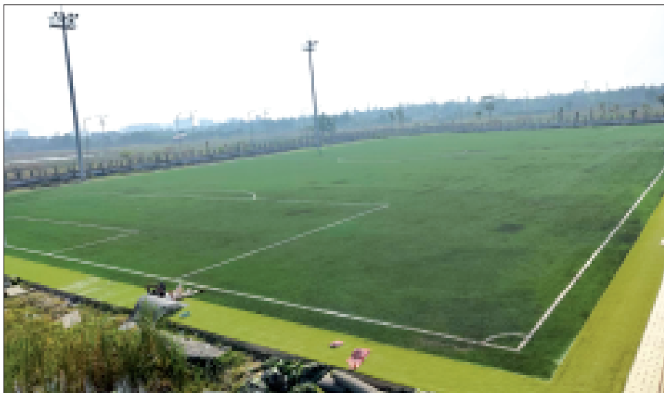
General View of Artificial Football Turf at NCE
